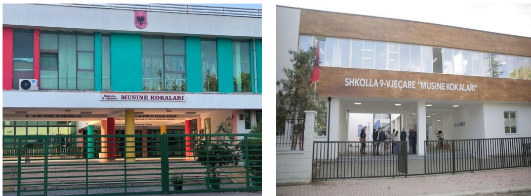
Fig.1 M.Kokalari school, before and after reconstruction
