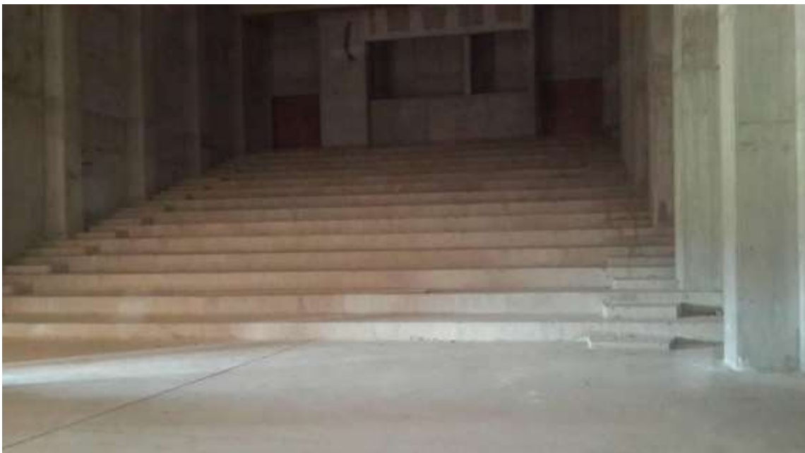
Figure 30 View from Conference Hall 2, under construction
