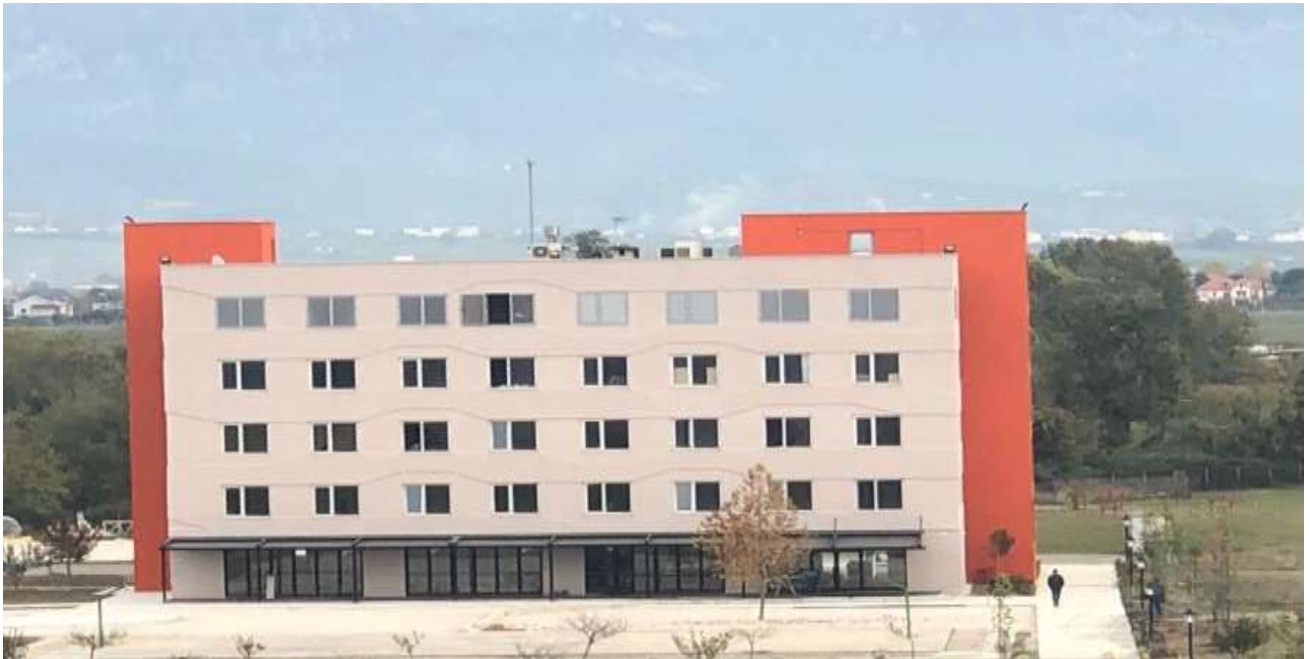
Figure 13: View of D-building
