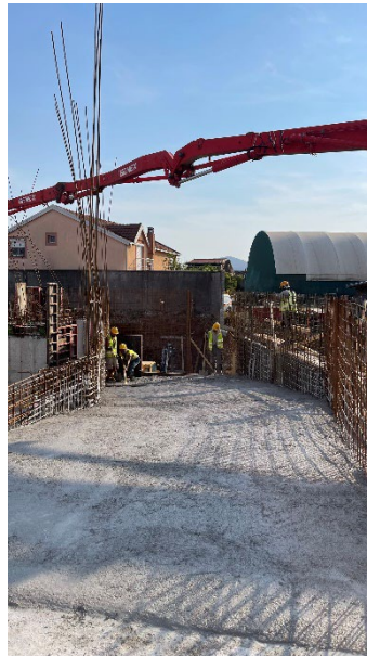
Figure 57 - Concreting Slab POS101-4
