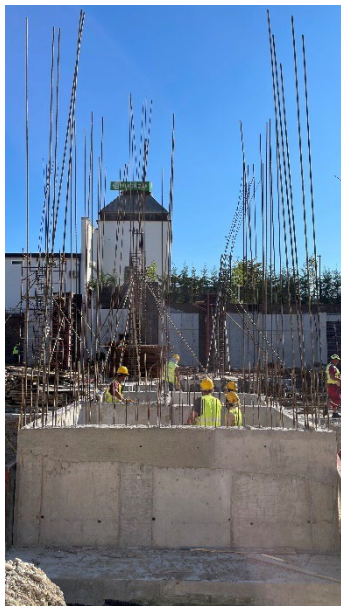
Figure 20 - Parapet Walls after removing formwork
