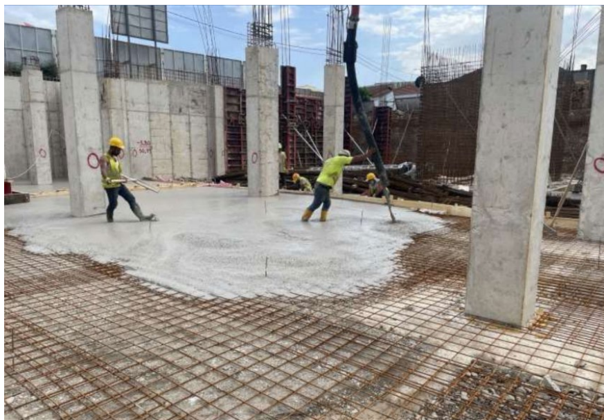
Figure 38 - Concreting the Garage Slab
