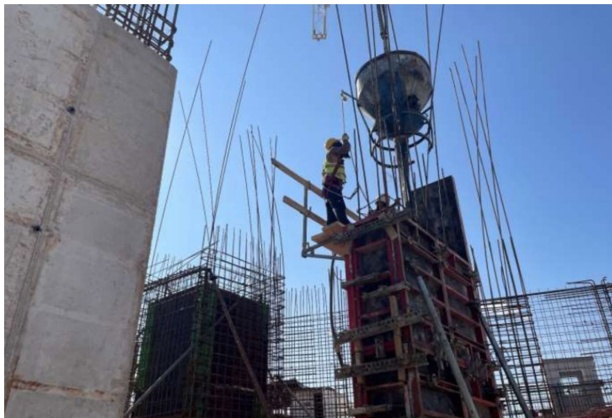
Figure 45 - Concreting Wall Panel POS Z-E-3
