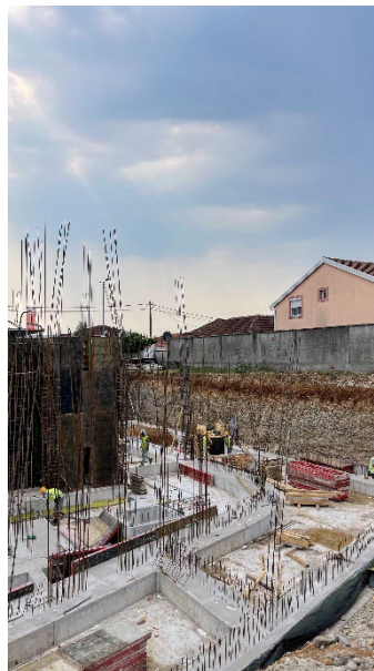
Figure 35 - Connecting Beams and Strip Foundation after being concreted
