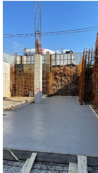
Figure 62 - Levelled Garage floor slab
