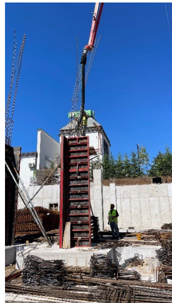
Figure 21 - Concreting the Columns
