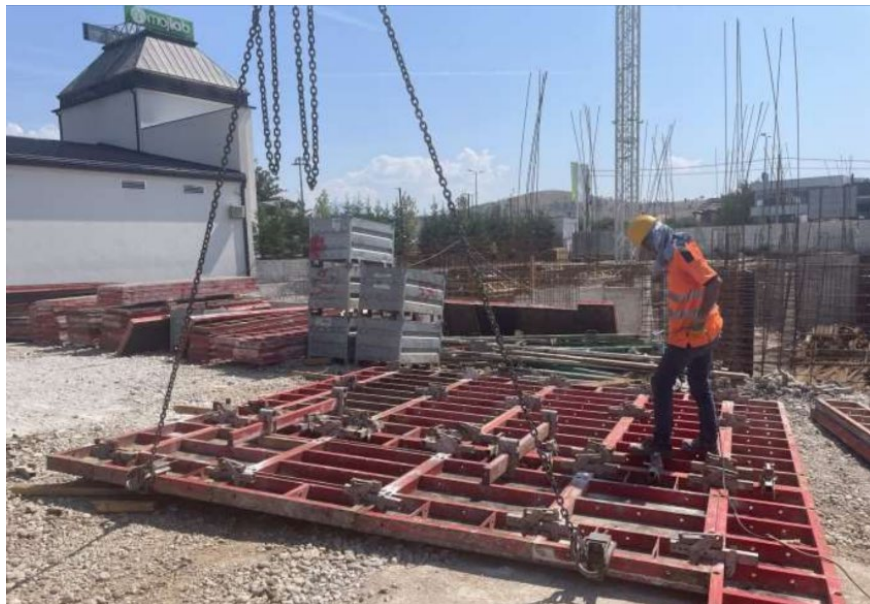
Figure 42 - Disassembly of Formwork
