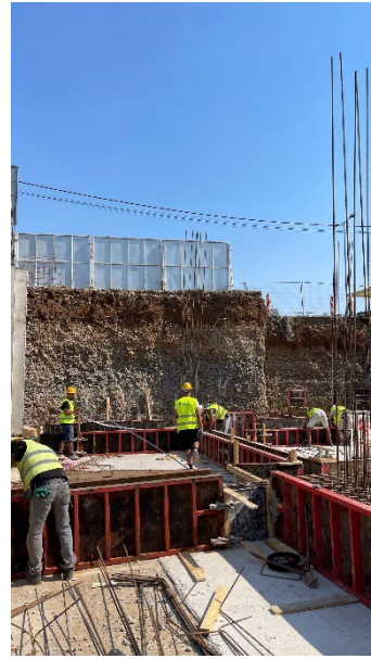
Figure 30 - Connecting Beams
