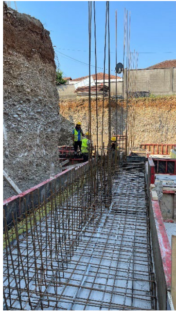
Figure 29 - Strip Foundation reinforcement
