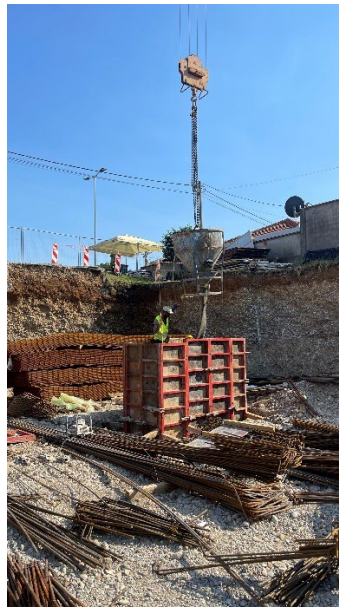
Figure 10 - Concrete pouring for Oil Separator Walls
