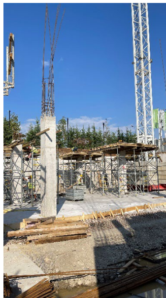
Figure 39 - POS100 Floor Slab Formwork
