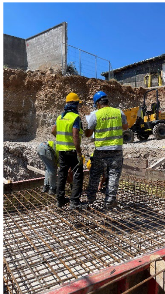
Figure 24 - Formwork and Reinforcement for Elevator POS Tp-3
