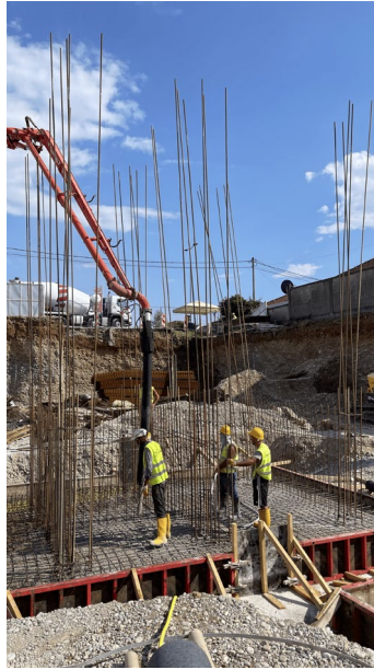
Figure 5 - Concrete pouring for the Elevator Foundation
