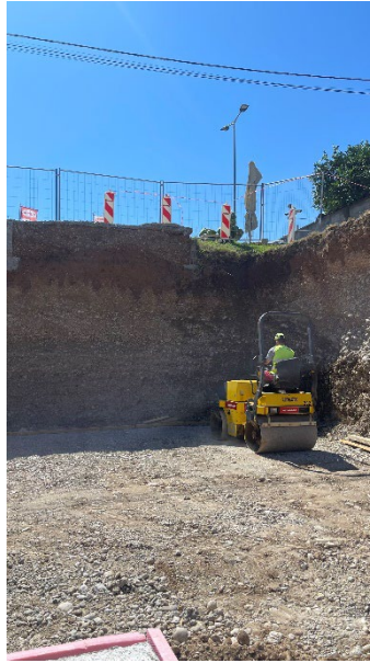
Figure 17 - Roller Compacting the Base Material
