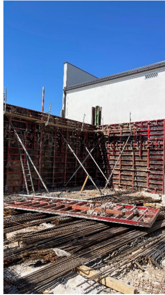
Figure 23 - Formwork of Walls
