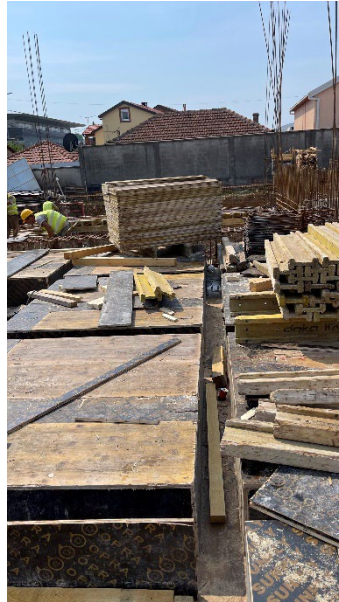
Figure 65 - Preparation works for POS100 floor level
