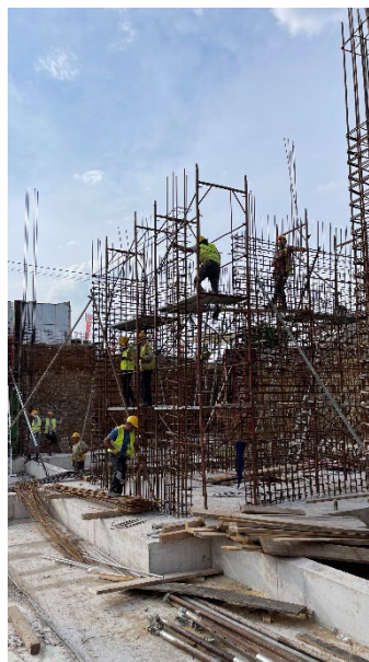
Figure 36 - Reinforcement work
