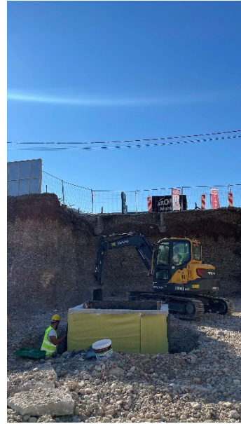
Figure 19 - Waterproofing of Separator
