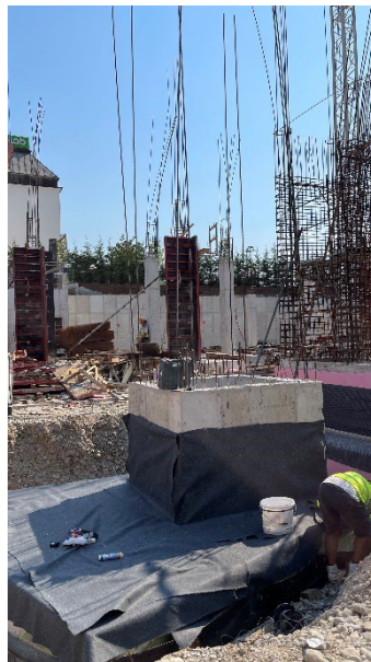
Figure 27 - Waterproofing System
