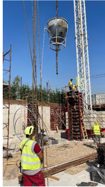
Figure 9 - Concrete Pouring for Column H,3
