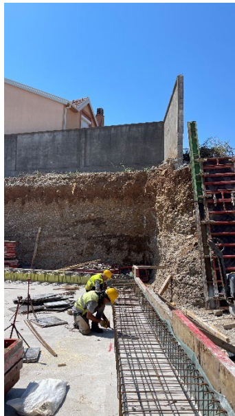
Figure 31 - Strip Foundation work
