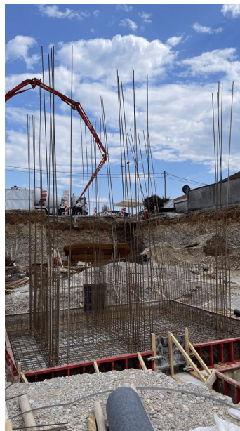
Figure 3 - Elevator Foundation
