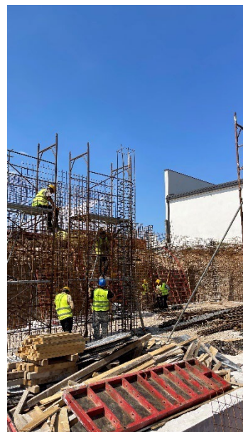
Figure 15 - Bar Reinforcement of Walls
