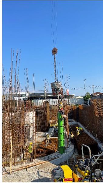
Figure 41 - Concreting Column S-7*
