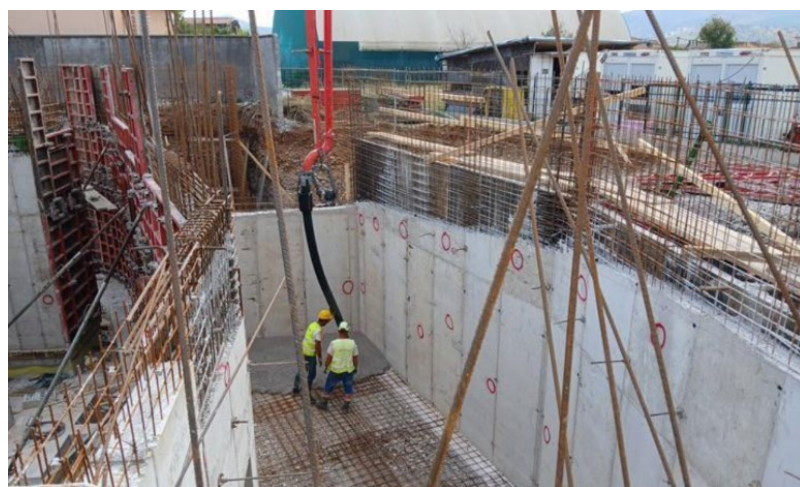
Figure 55 - Floor slab concrete pouring
