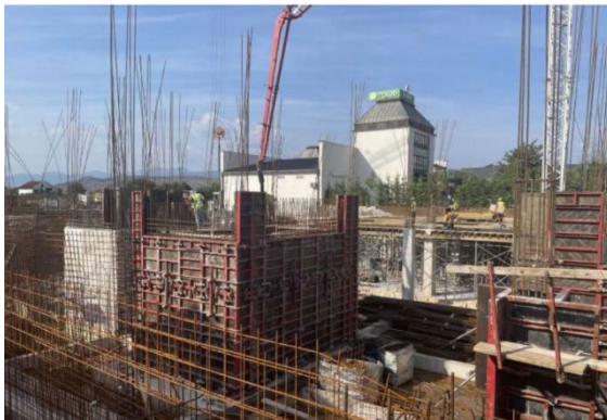
Figure 43 - Concreting Walls
