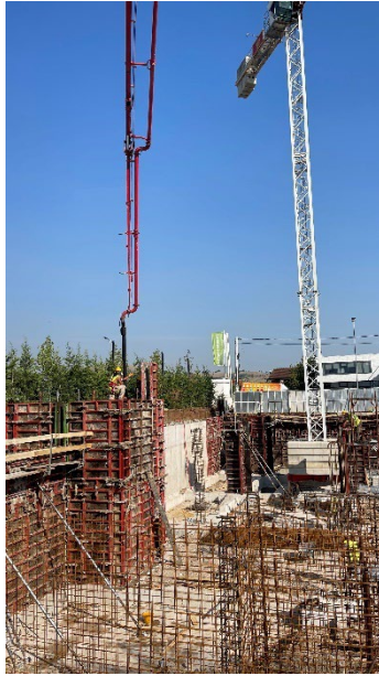
Figure 8 - Concrete Pouring for Specified Walls
