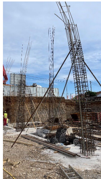
Figure 12 - Reinforcement of Columns
