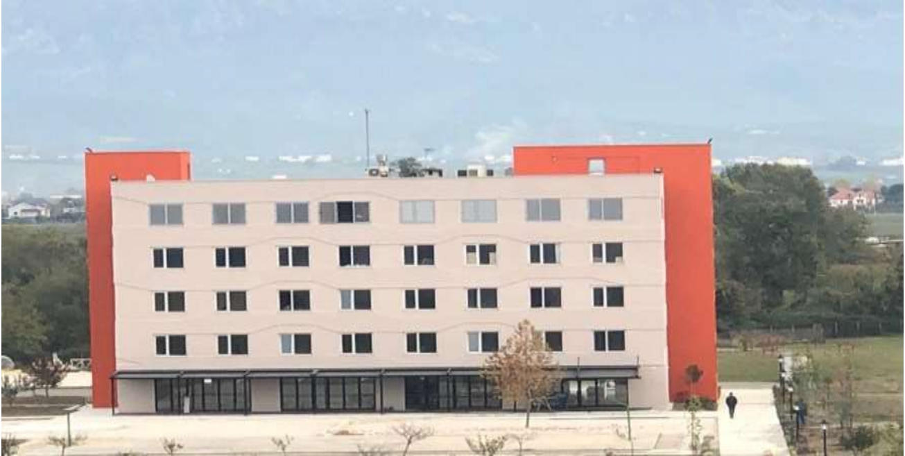
Figure 13: View of D-building
