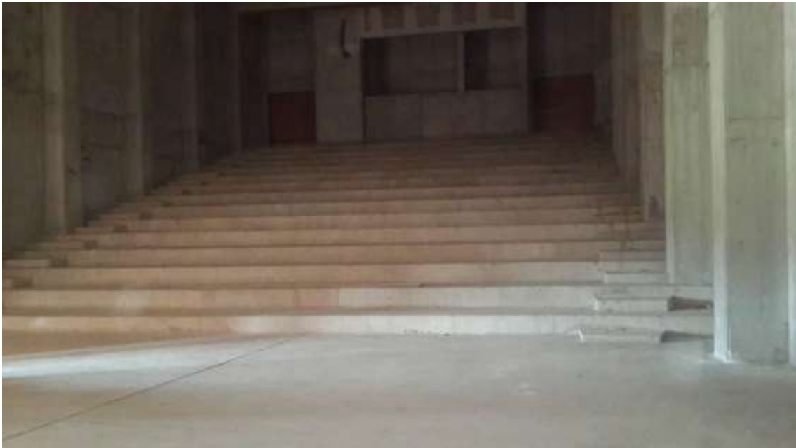
Figure 30 View from Conference Hall 2, under construction
